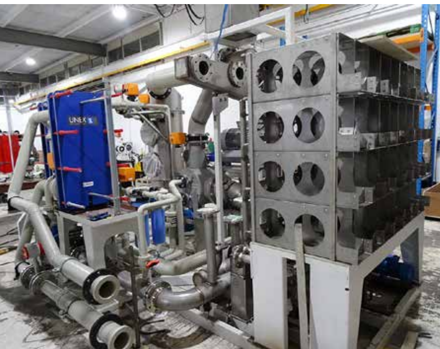
Fabrication of the fuel cell for the FPS Maas.
