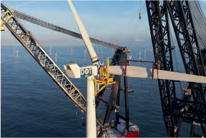
Heerema's GREPT in action (photo Heerema).
