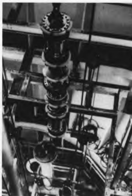
fig. 10: RPIT hoisted over J-tube in platform leg
