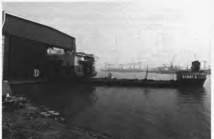
fig. 32: Load-out operation in progress
