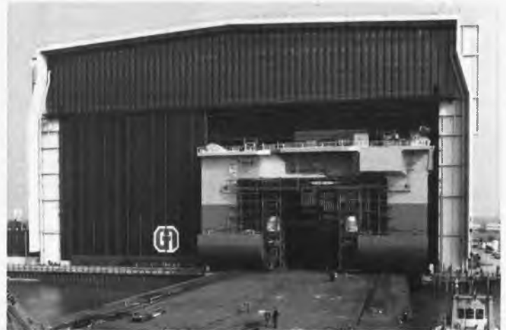
fig. 31: Giant 2 submersible barge in way of Smit Semi I
